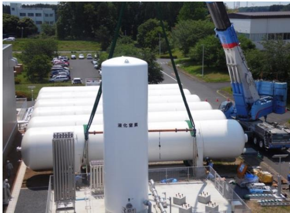
JT-60SA Helium Storage Vessels Final Assembly
